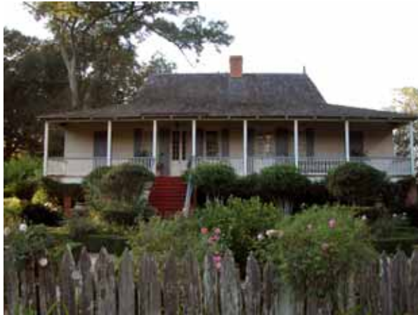
This Creole Cottage exhibits the simplicity of farmhouse massing, with un-composed column spacing and windows and doors that do not align with column openings.
