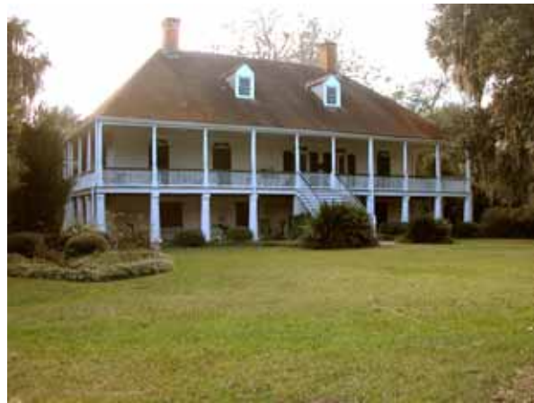
This 1750 Creole Plantation is the classic of its type. The pavilion roof, raised basement, gable dormers, interior fireplaces, and galleries are all iconic examples of this style.
