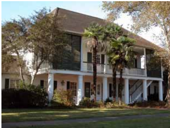
This Creole Plantation has massive masonry columns at ground level and an exterior gallery stair leading to the level above.
